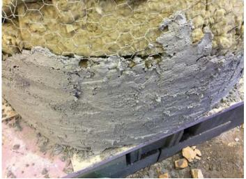
Let oven dome sit overnight then remove sawdust and newspaper with a small garden hoe. Keep oven damp and covered with plastic for 7 days to cure mortar. Start small curing fires to dry out any excess moisture.
