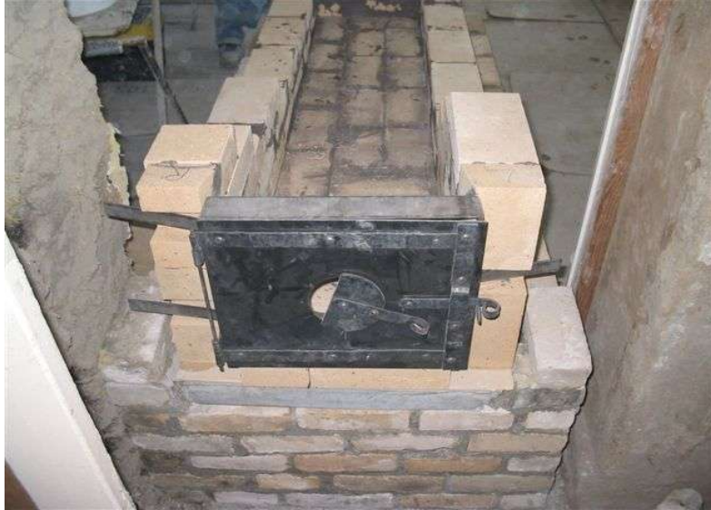
Additional views and from kitchen showing replica inner loading door.
