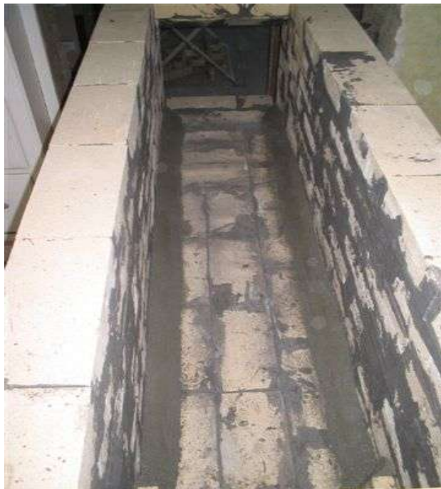
Firebox view before setting ceiling. We created a poured in place floor slope with castable since we felt the firebox being too narrow to accommodate a 45Deg. half firebrick. We did use firebrick cut at 45deg. At the far end of the firebox. Another view from front without loading door.
