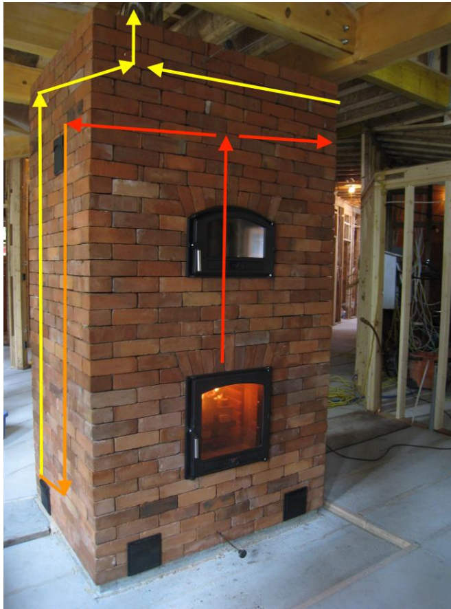
Figure 4: Superimposed arrows showing flow direction on an actual unit.
