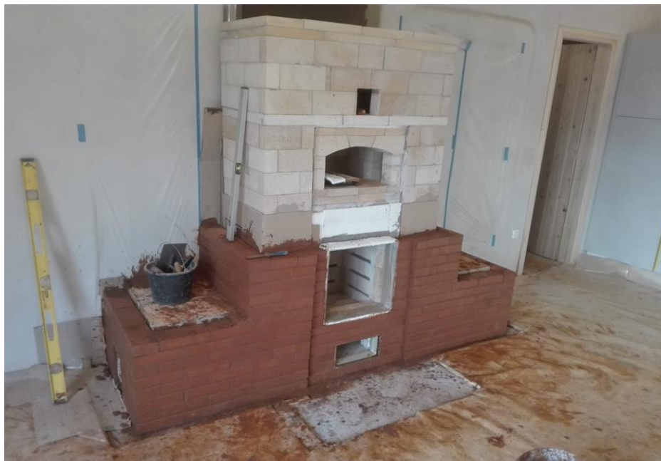
Figure 6: The 'Core' of the heater constructed of firebrick and refractory mortar is separated from the 'Skin' of the heater by cardboard and ceramic fibre.
