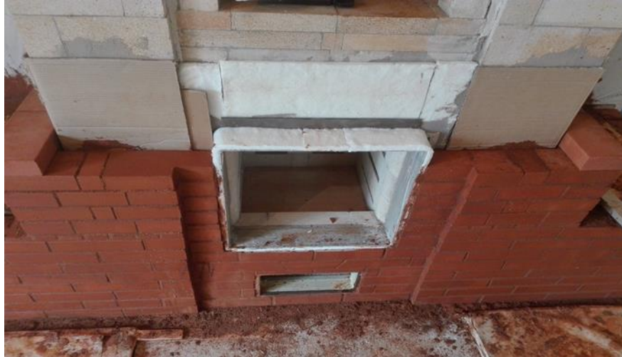
Figure 7: The entire 'Core' of the heater is completed prior to facing the heater. Note: clean outs are visible on the side of the bench as well as below the firebox and above the oven.
