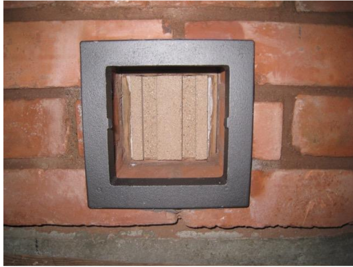
Figure 5: Cast iron clean out frame door not attached)- fire brick plug in core.
