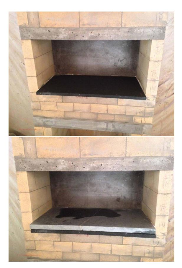
For our firebox lintels we have been using a piece of  $1/8" \times 2.5" \times 4.5"$  stainless steel bent into an angle iron L shape laid down over the opening and then we set a piece of 1/4" high temperature painted mild steel angle iron on top of the stainless steel. It is a simple and fairly inexpensive method that has been in use for us since about 2006 with no warping or failures.
