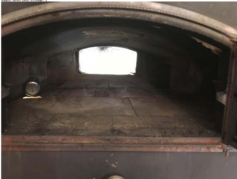
Lower deck (note the plate covering the coal chute)
