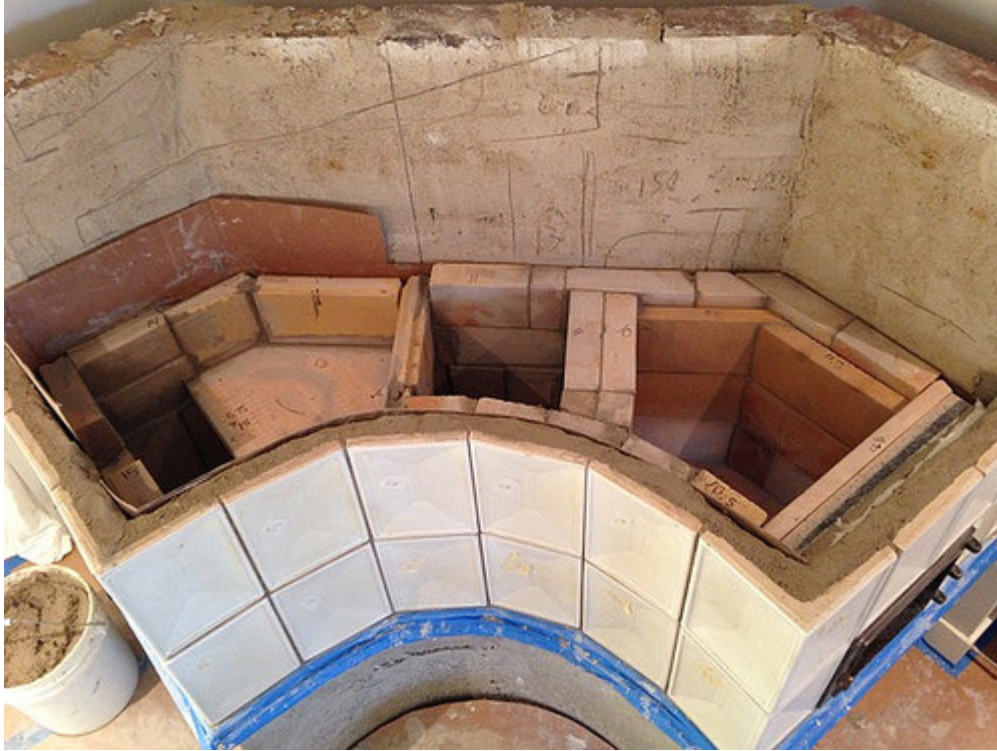
Austrian Kachelofen or Tile Stove showing the Engine or Core of the unit with some of the channeling.
