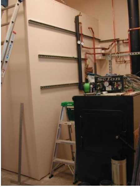
Figure 3. CCHRC wood-fired hydronic heater with 1,400 gallon thermal storage tank.
