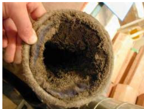
Figure 12 regular replacement of filters is important for IAQ, source: AEE Institut für Nachhaltige Technologien
