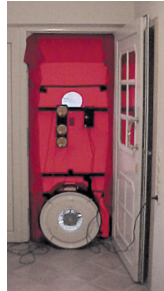
Figure 7 Blower-door-test Source: www.passivhaus.de
