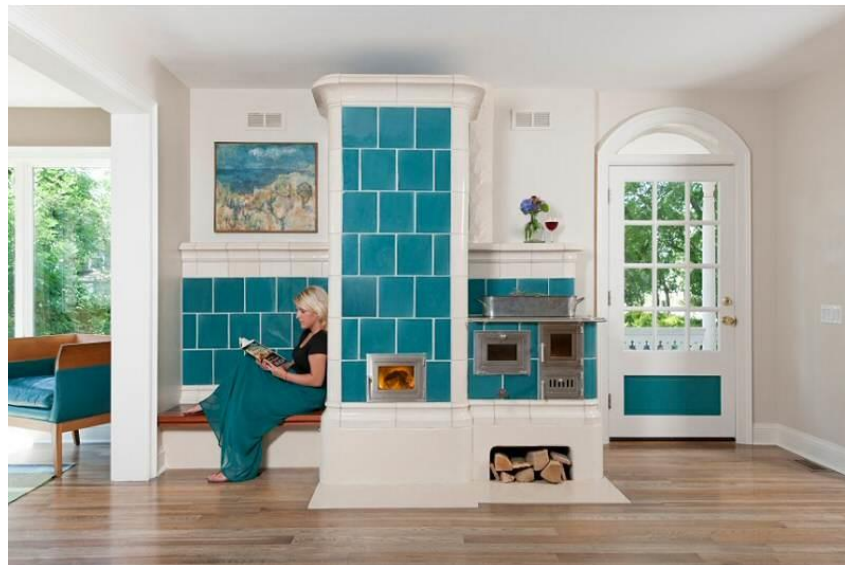
Example of Austrian inspired Kachelofen style masonry heater custom built and site assembled
