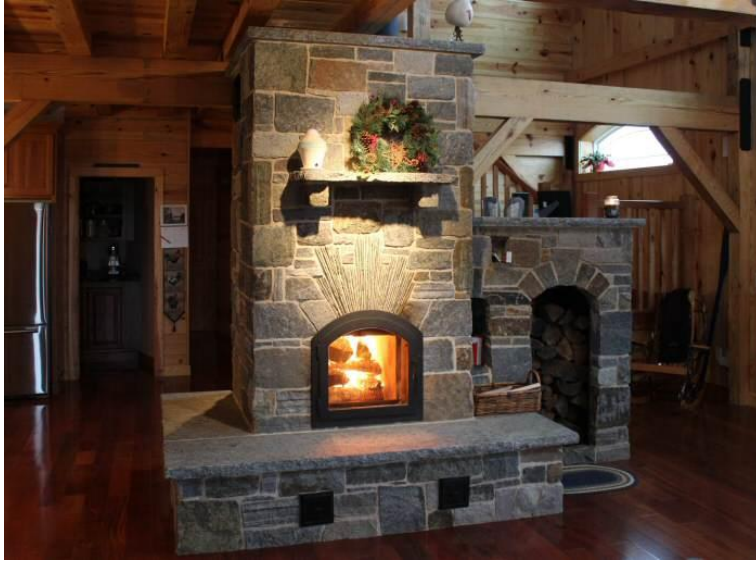
Example of site-built masonry heater with manufactured core system and assembled on site
