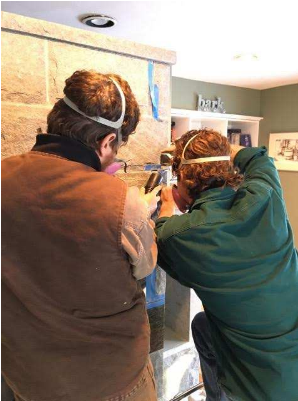
and gouge out the pieces. Mason and his helper took turns with the vac and the grinder.
