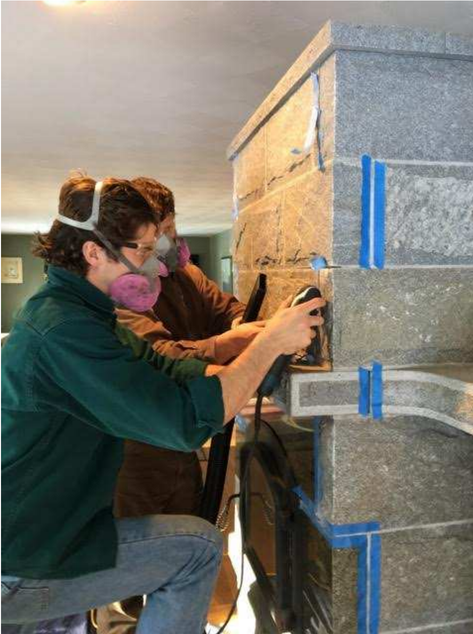
The tape also kept the stone clean during tuck pointing.
